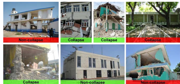
Figure 1. collapse classification results. Note that text labels indicate classification results and green and red colors are true and false estimation.
