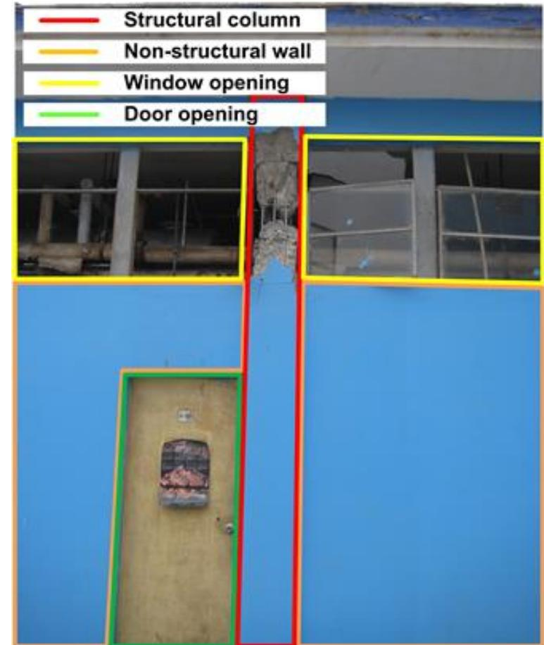
Spalling on a captive column
